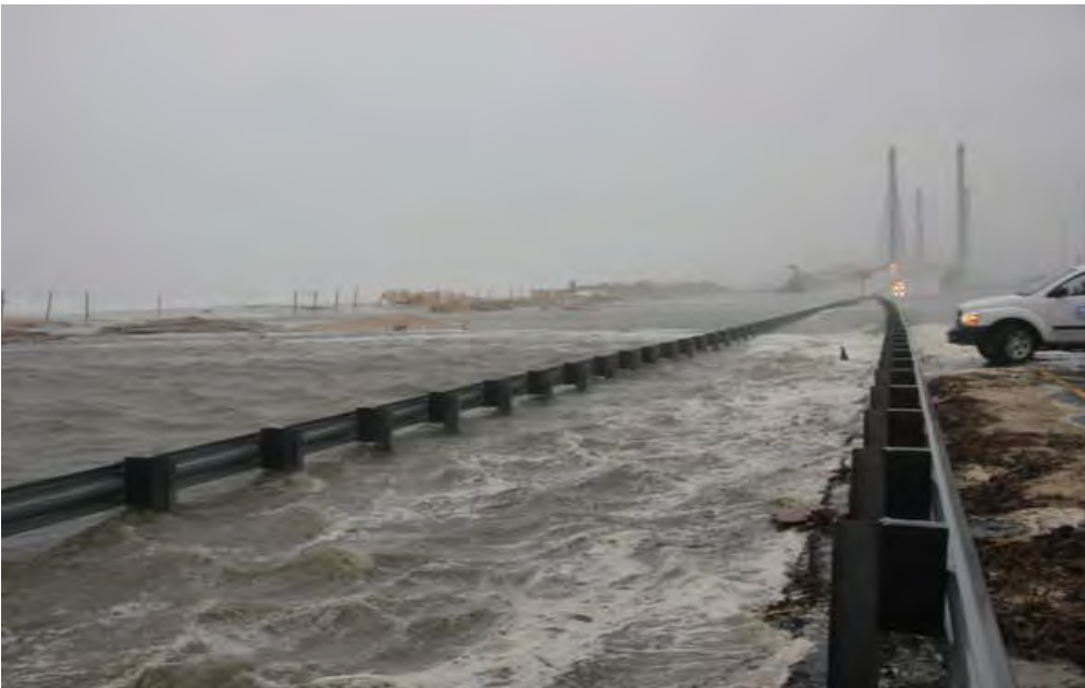
Photo 2: State Route 1 and Indian River Bridge during a recent storm (water pooling) (March 6, 2013).
